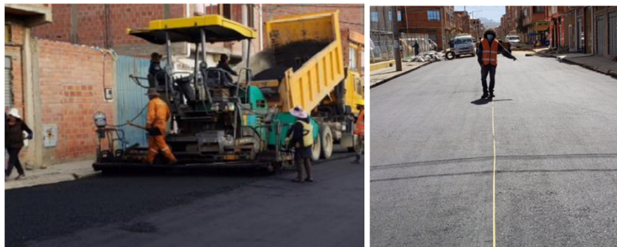
Figure 7: Test Road construction.
