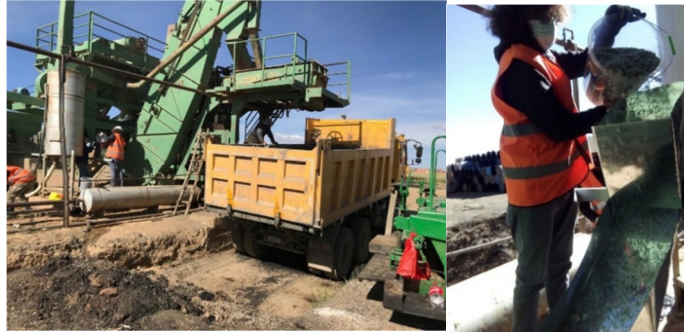
Figure 6: Addition of PET to asphalt mix in plant.
